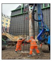
• 60% of the Secant pile guide wall is complete which allows for the secant pile installations to commence.
