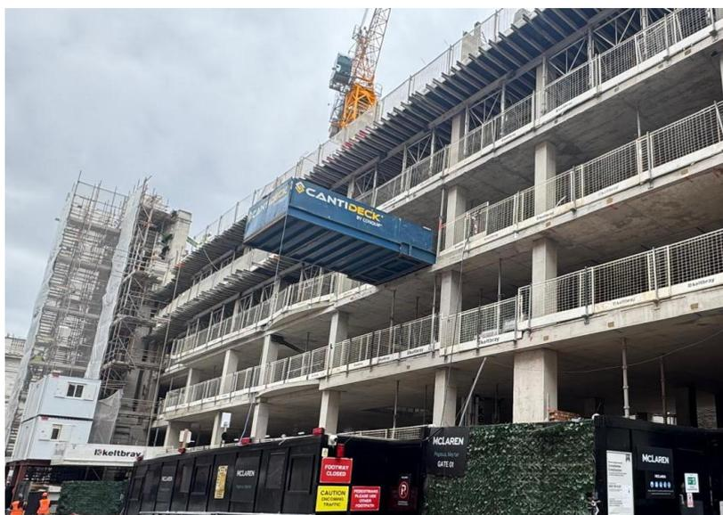
In the last period, the site logistics plan has transitioned to the next phase. Within the month of April, tower crane two was erected and tower crane one dismantled. A goods hoist now services ground floor to level three, with further capacity aided by two cantidecks on Sackville Street.
