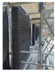
We are extremely pleased to communicate that the removal of the façade retention system (green steelwork) has started. The steelwork was essential to support the façade during demolition and the construction of the new concrete frame. It is a key milestone of the project to reach this point where the building façade is returned to its original state.
